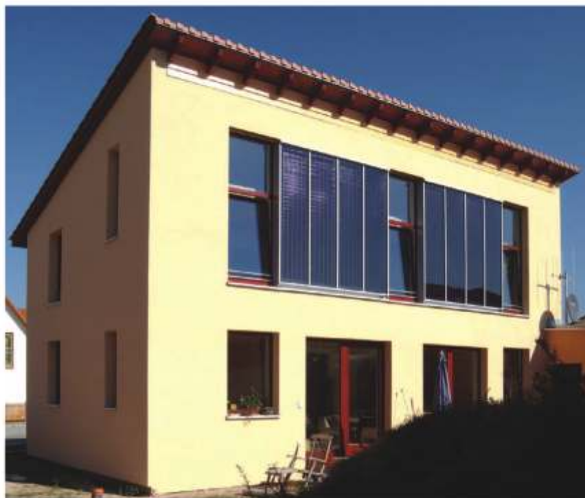
Fig. 2-29: Exemplu al unui colector de fatada FK REHAU-SOLECT
